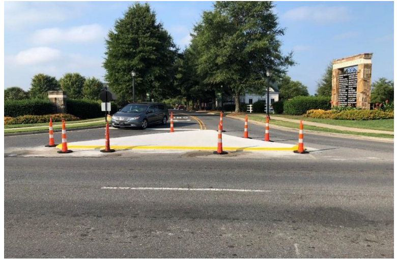
Access Management Improvements at Baxter Village Town Center and SC 160
