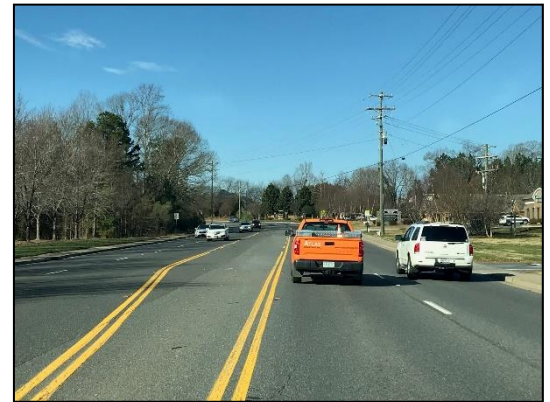
Example of a minor arterial: Gold Hill Road
