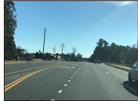
Example of a principal arterial: SC 160
